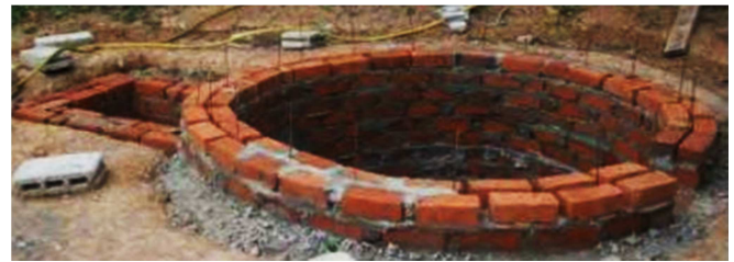
Figure 3. Installation of biogas plant.
