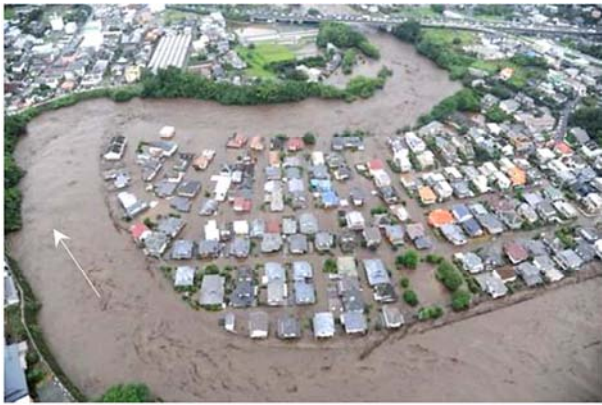
Figure 1. Flood of July 2012 at the Shirakawa River.
