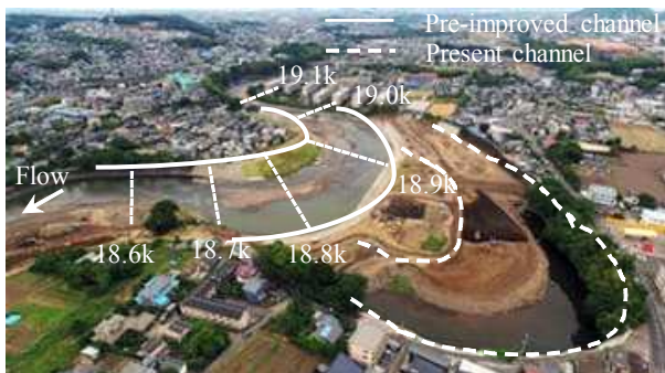
Figure 2. New channel of the Shirakawa River.
